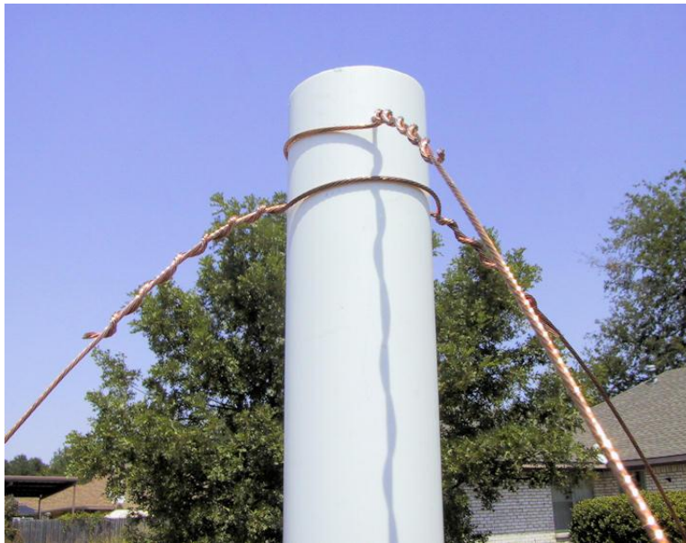
Figure 2: Attachment of wires to mast.
